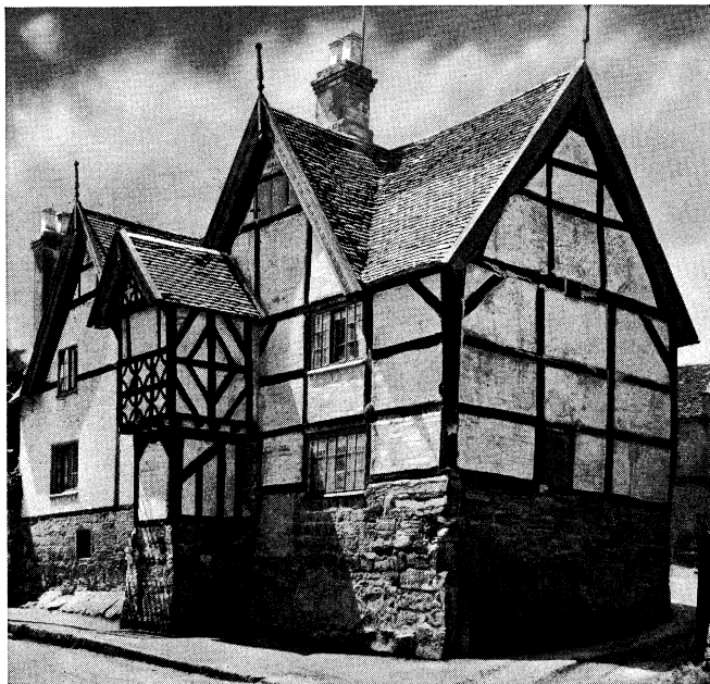
Chantrey house, Castle Donington, Eng., gabled half-timber house of the 16th century
